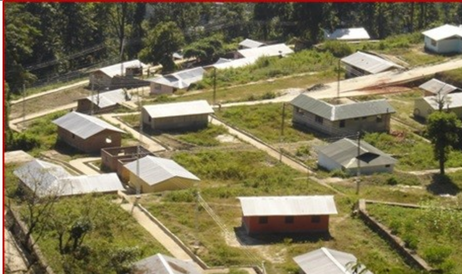
Fig.5.11: View of Resettlement Colony at Teesta-V Power Station, Sikkim
